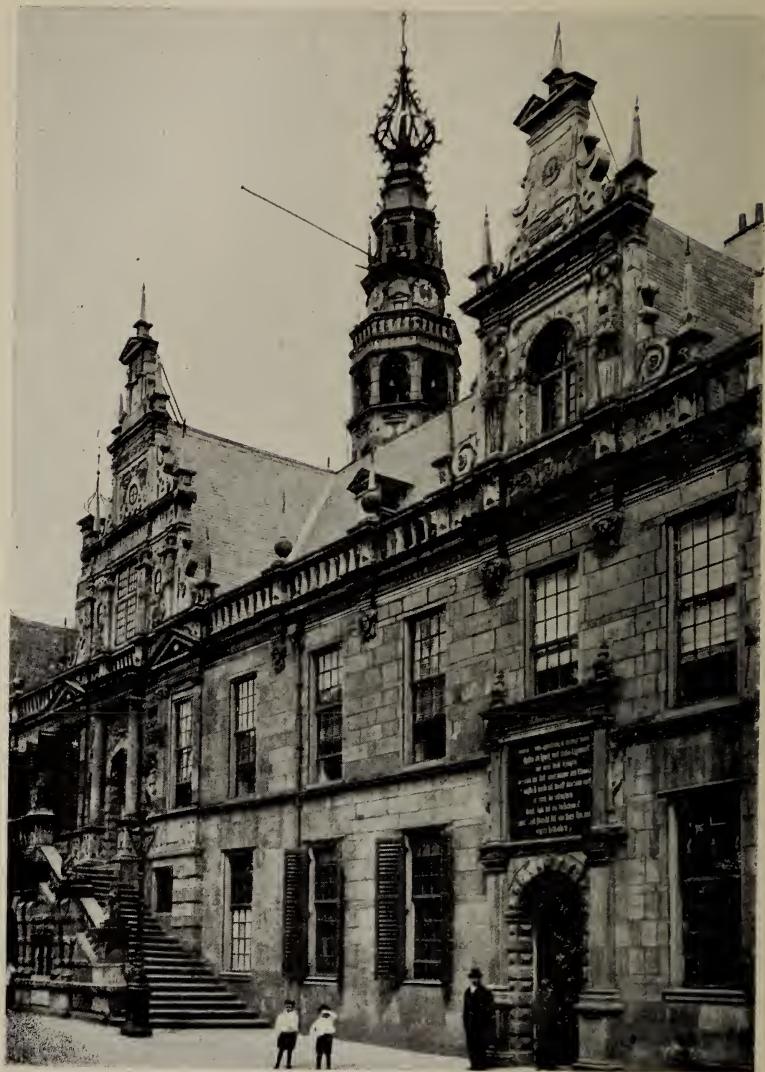
LEIDEN: THE TOWN HALL CARILLON TOWER
